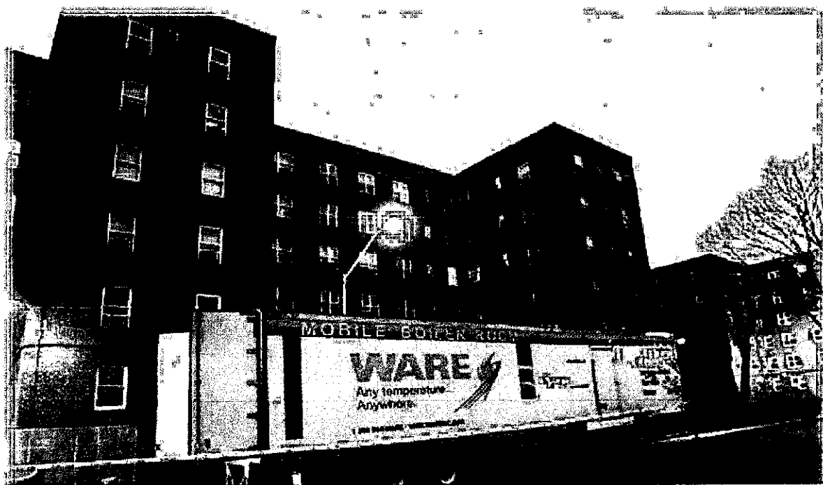
Figure 10: Several buildings of the Red Hook Houses remained without electricity, heat or hot water weeks following Hurricane Sandy. While power has been restored, trailers like the one above have remained. Residents want them removed (NYCHA)
