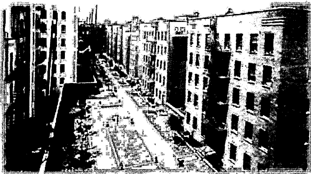
Figure 3: Workers put the finishing touches on First Houses, the City's first public housing development on New York's Lower East Side, 1935. (NYCHA)
