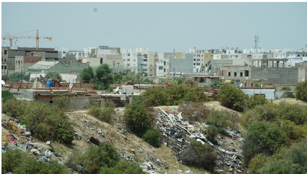
Figure 1: Outskirts of a growing neighborhood in the south of Tunis. Industrial waste from construction can be found wherever new houses are built.
